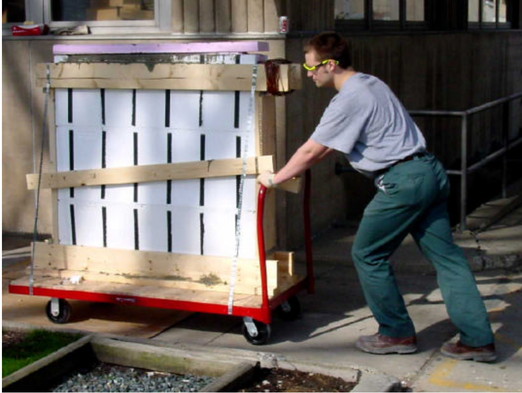
Figure 2. ICF wall section were constructed on a movable carts.
