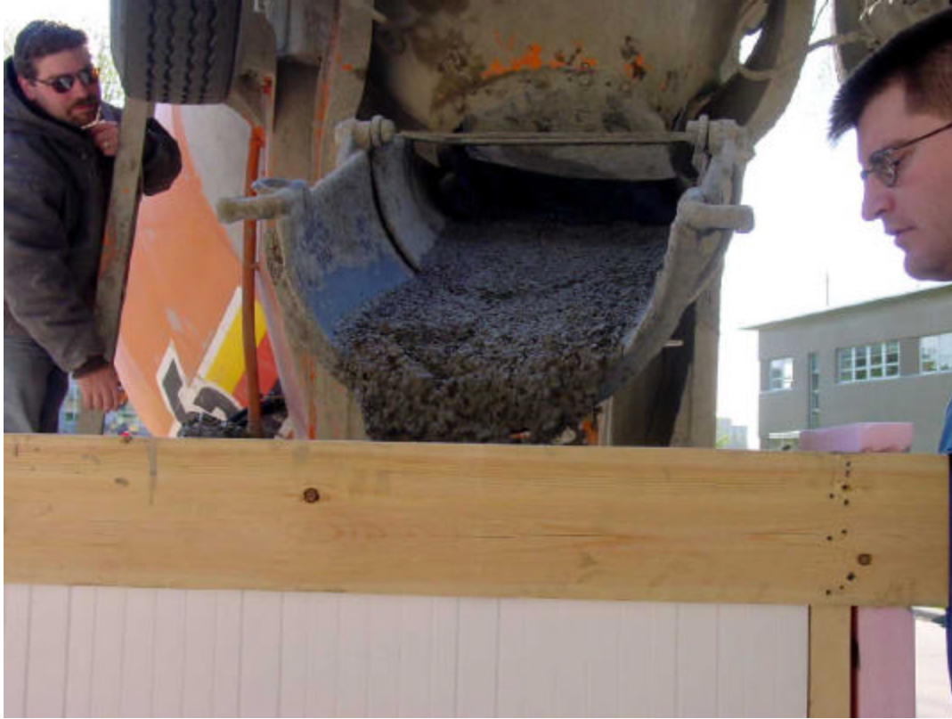
Figure 3. Concrete was placed directly from ready-mix truck into wall sections.
