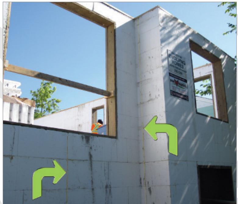
Here is a job, post concrete, that has been constructed exactly to the building dimension by properly stacking seams.
